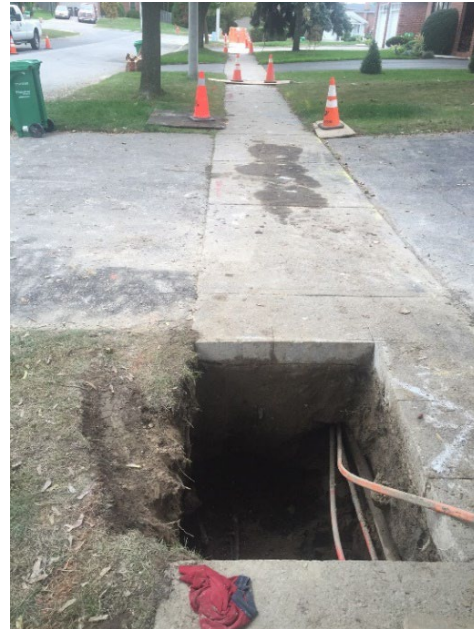
Figure 10: Excavated direct-buried XLPE under a sidewalk
