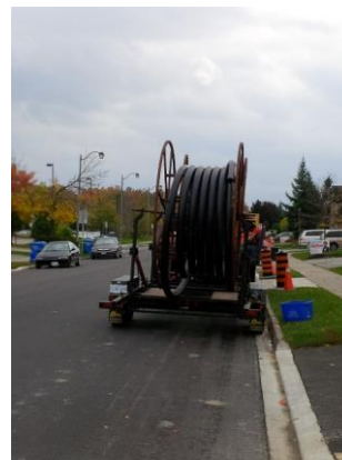
Image: Cable truck parked in residential neighbourhood
