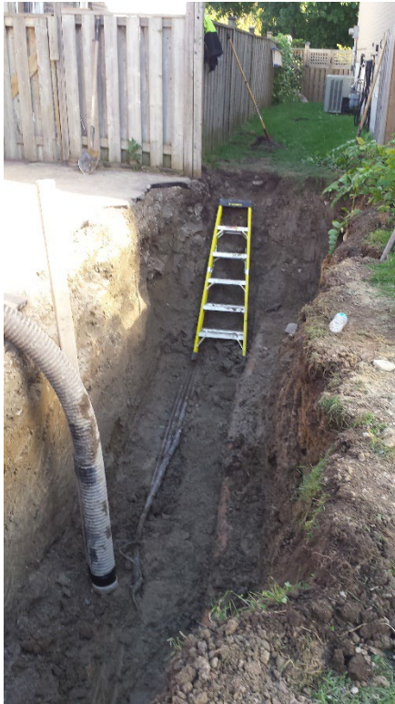
Figure 20: Excavating direct-buried XLPE cables in a residential rear-lot
