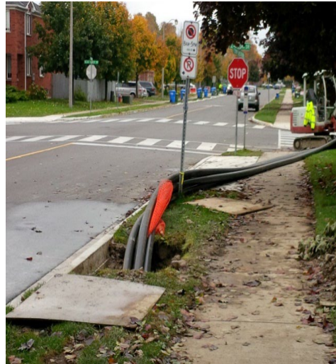
Figure 13: Installation of new cable in duct
