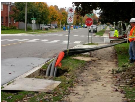
Image: Cable-duct being installed along a residential street
