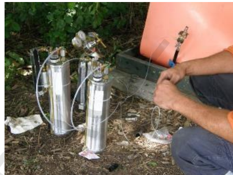
Image: Cable injection preparation
