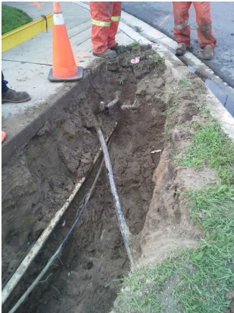
Figure 9: Excavated direct-buried XLPE Cable
