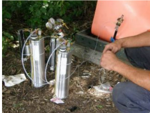
Figure 11: Application of cable injection fluid
