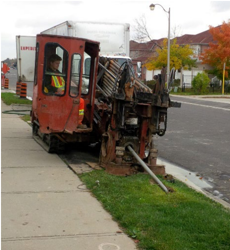
Figure 12: Direction Bore Machine installing new duct for cable replacement
